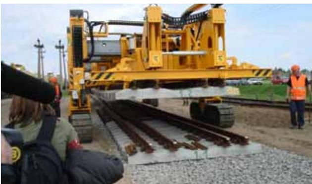
Laying the first of the new dual 1,435/1,520 track sections on the "Rail Baltica" line at Sestokai, Lithuania
