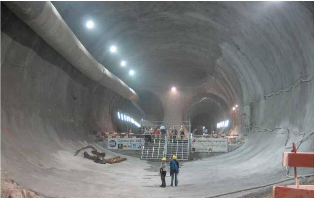
Y-junction (TV-WS, Tunnelverzweigung West-Süd) in the western tube of the Gotthard Base Tunnel at Multi-Function Station Faido, Canton Ticino, Switzerland.
